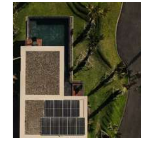
THE VICTORY BY ANDAMAN ASSET SOLUTION
